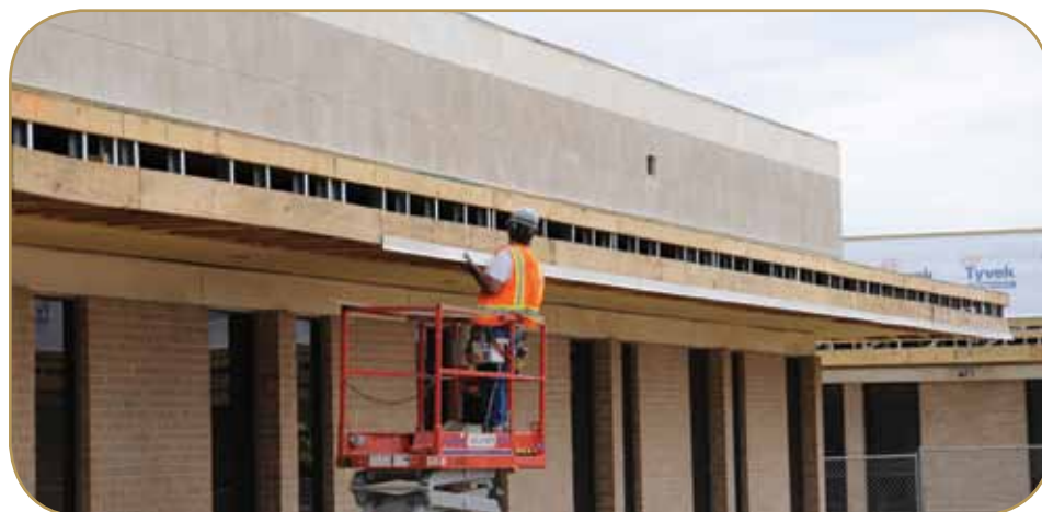
Upper photo: An artist's rendering of WC's new academic building (courtesy of Hahnfeld Hoffer Stanford). Lower: A construction worker placing metal trim on the Biology Building mansard.
